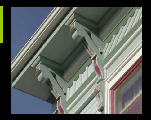
A corbel is a bracket made of stone or wood which juts out from a wall and is used to support an oriel window, a balcony or a roof cornice.
