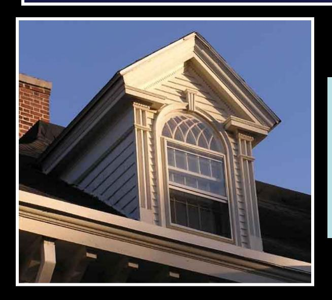
A window set vertically in a small gable projecting from a sloping roof
